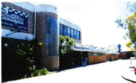
Figure 2: Existing buildings on site.
